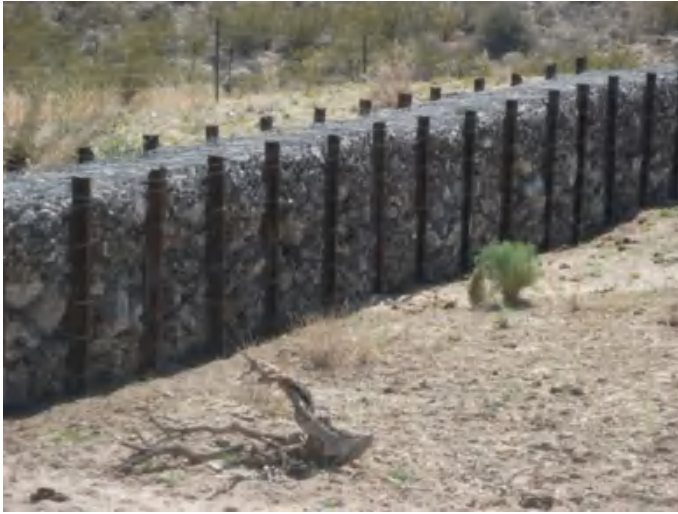
Fig. 16.6 Gabions used for ephemeral stream bank erosion control, northwestern Arizona
