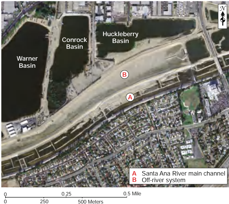
Fig. 15.13 Santa Ana River, Orange County, California, in-channel and off-channel recharge facilities. A series of low berms in the main river channel (A) create a more tortuous and slower flow. Off-channel recharge basins parallel the main channel (B) and are present further to the north (Source U.S. Geological Survey)
