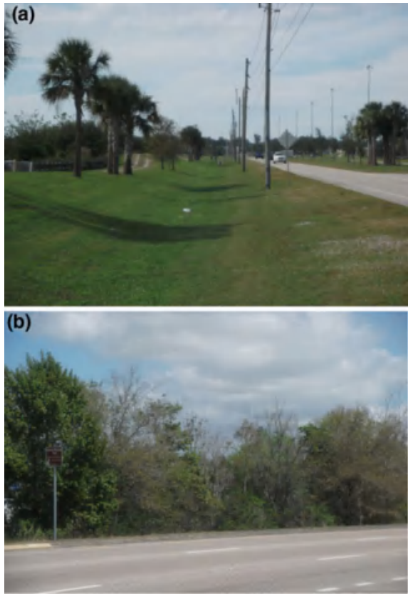
Fig. 23.1 a Grassed dry swale, Sarasota, Florida. b Wet swale (treatment wetland), median of Daniels Parkway, Lee County, Florida
