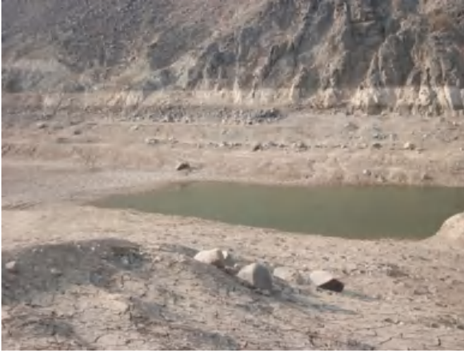
Fig. 16.8 Mud-cracked recently deposited sediments in the Murwani Dam reservoir, western Saudi Arabia
