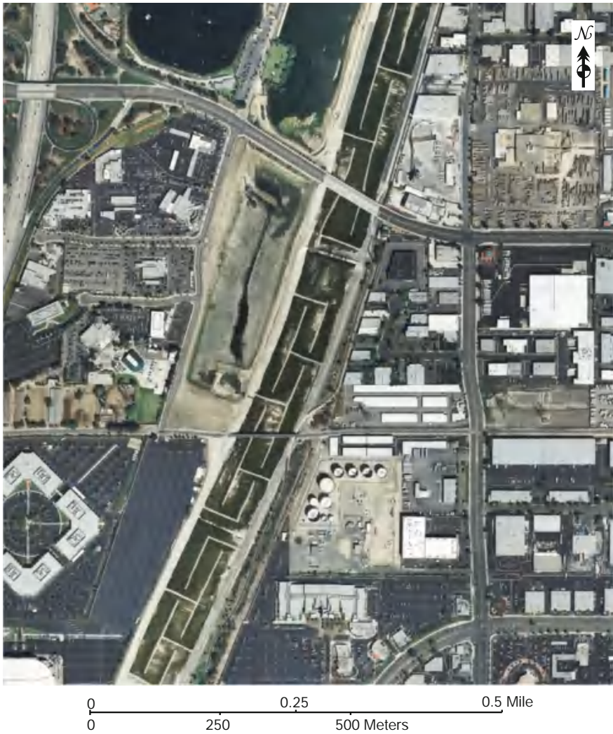
Fig. 16.3 Temporary in-channel levees in the Santa Ana River, Anaheim, California (March 28, 2010, source U.S. Geological Survey)
