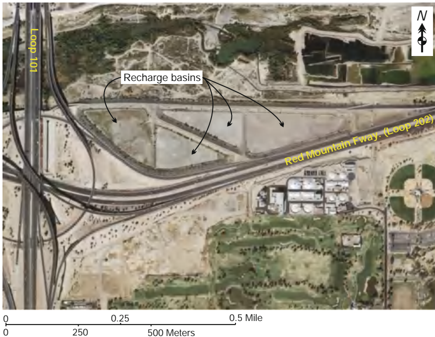
Fig. 19.3 Aerial photograph of the Mesa Northwest Water Reclamation Plant SAT system, Arizona (Photograph source: U.S. Geological Survey)
