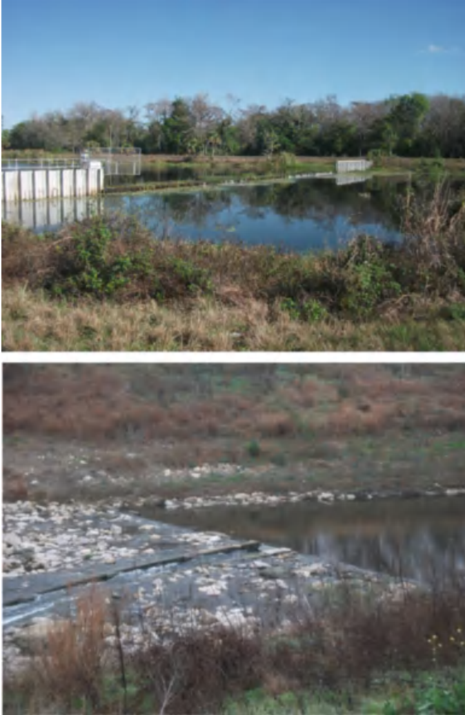
Fig. 16.5 Weirs. Top: South Florida Water Management District West Weir, Seminole Tribe of Florida Big Cypress Reservation. Bottom: San Antonio River, San Antonio, Texas
