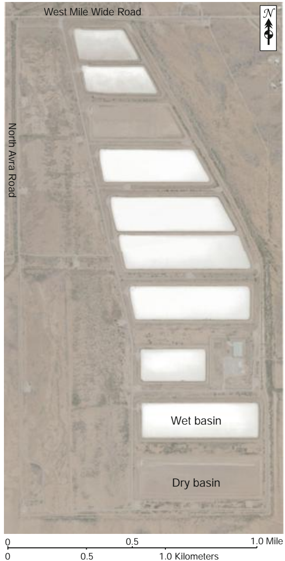
Fig. 15.12 Aerial photographs of the Central Avra Storage and Recovery Project located near Tucson, Arizona (May 2015; Source U.S. Geological Survey)
