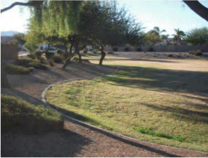
Fig. 15.6 Residential infiltration basin in Sunrise, Arizona, which was made to be a community amenity (playfield)
