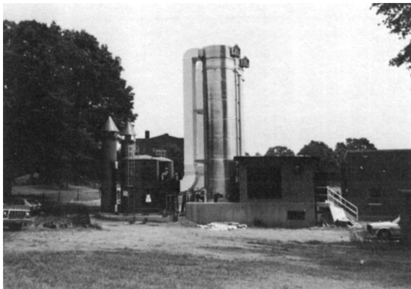
FIGURE 2-18. Packed-tower air stripper with VPGAC.
