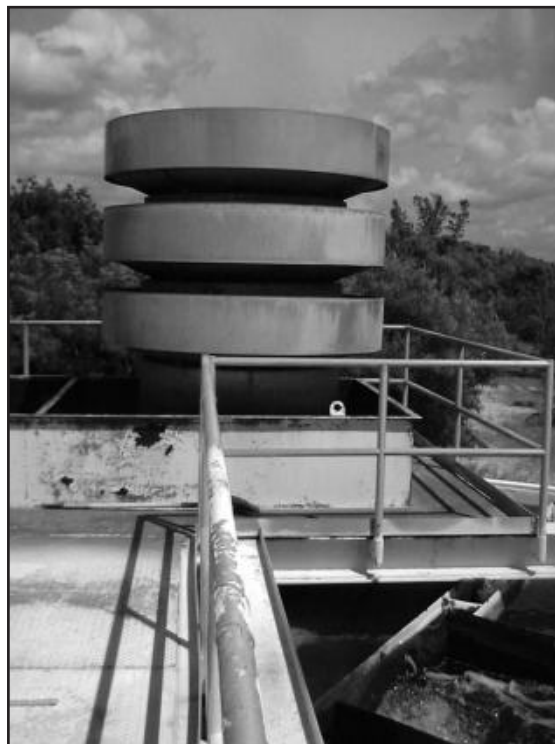
Figure 9-1 Natural draft aeration system
