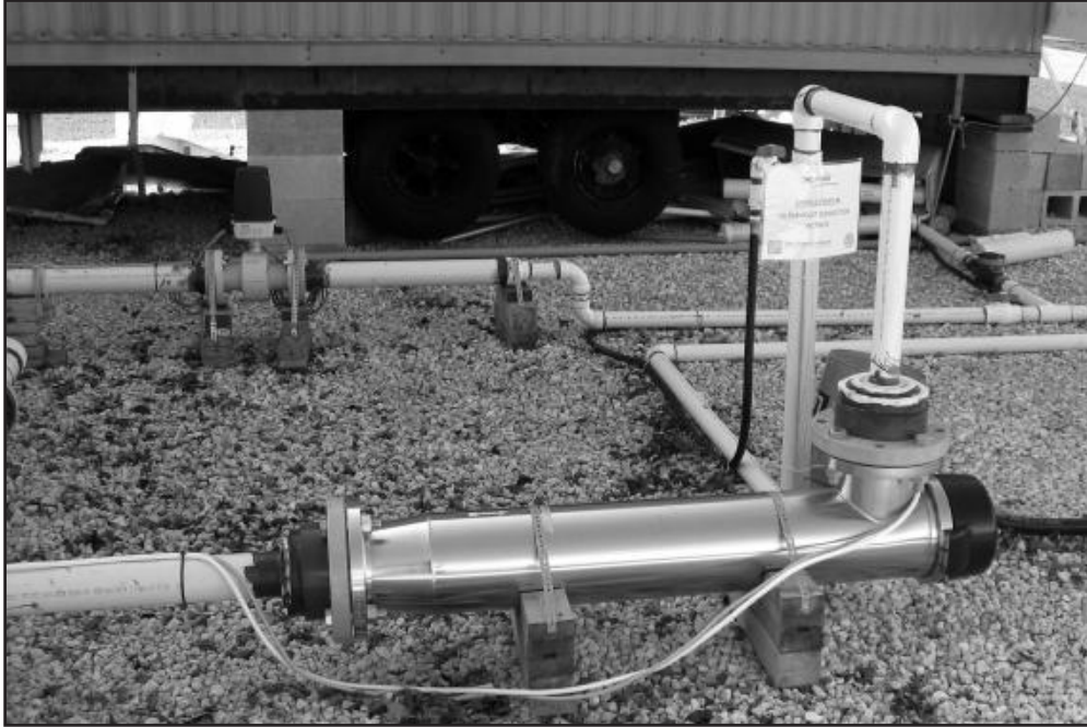
Figure 9-5 UV light system
