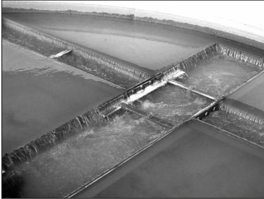
Figure 9-12 Example of filter being backwashed. Backwashing needs to occur regularly but the backwash should be recaptured to improve water use efficiency.
