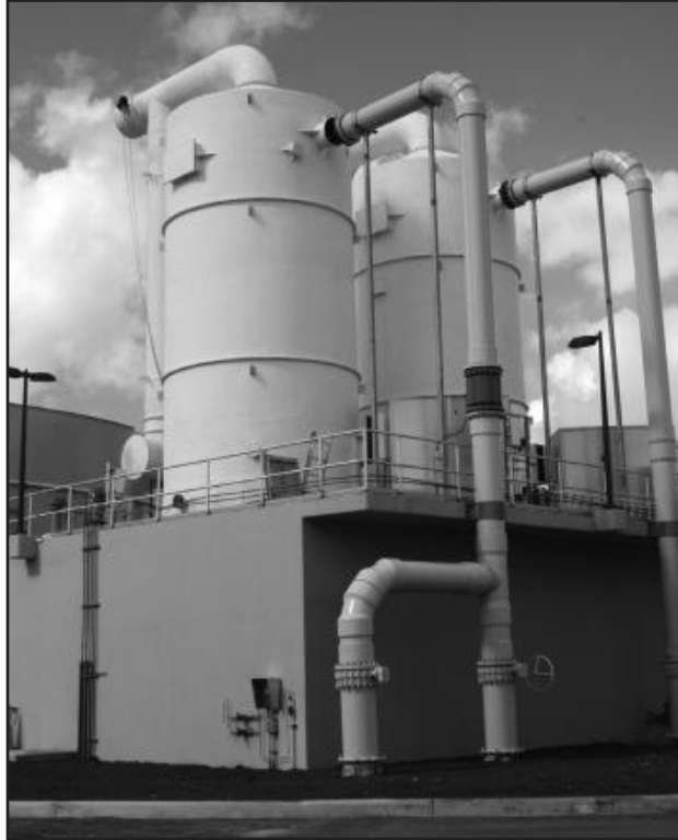
Figure 9-2 Packed-tower aeration
