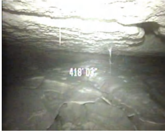
Fig. 18.6 Downhole video photograph of a paleokarst cavern, City of Sanford, Florida ASR exploratory well. Cavern is located approximately 127 m (418 ft) below land surface and 116 m below sea level
