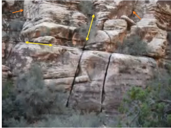
Fig. 17.2 Fractures in an eolian sandstone at Red Rock Canyon, near Las Vegas, Nevada. Sets of fractures parallel and perpendicular to bedding are clearly evident (yellow arrows). Other perpendicular or oblique fractures with different orientations are also evident (orange arrows)
