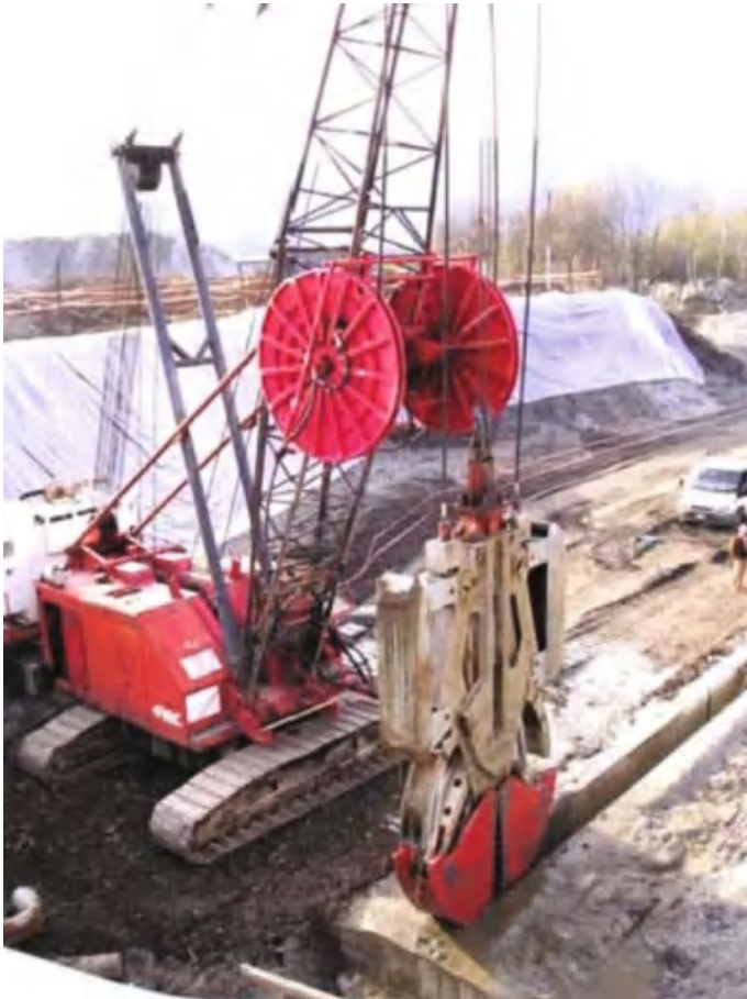
Fig. 17.38 Hydraulic clamshell-bucket crane used to excavate the barrier trench
